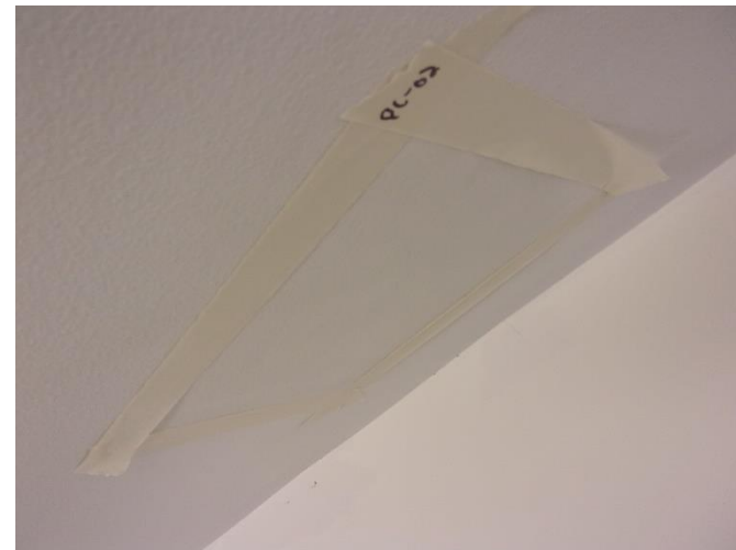
View of example sample location for post-cleaning sampling
