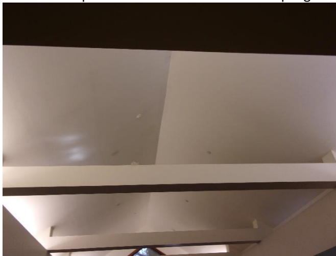
View of complaint area ceiling with no visible mold
