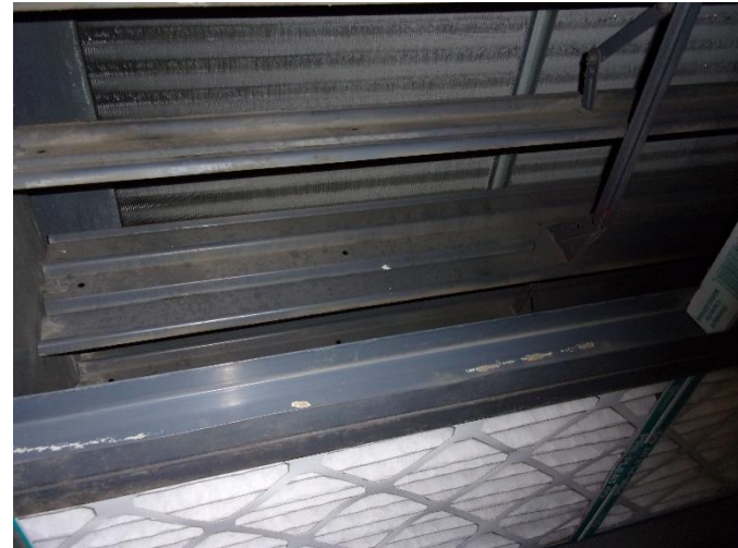
View of HVAC AHU on initial visit
